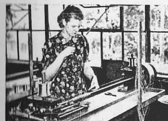
Every string made by Gibson is hand wound by girls long experienced in the work. Hand winding insures tightness of each loop, greater accuracy and strength, and longer wear.
